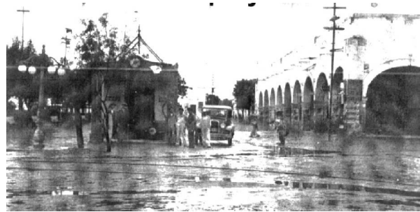
CASETA HUASTECA PETROLEUM COMPANY
